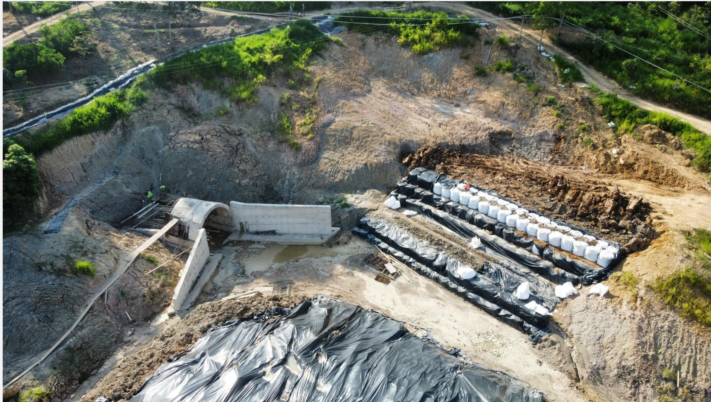
Portal Construction on January 23, 2025
