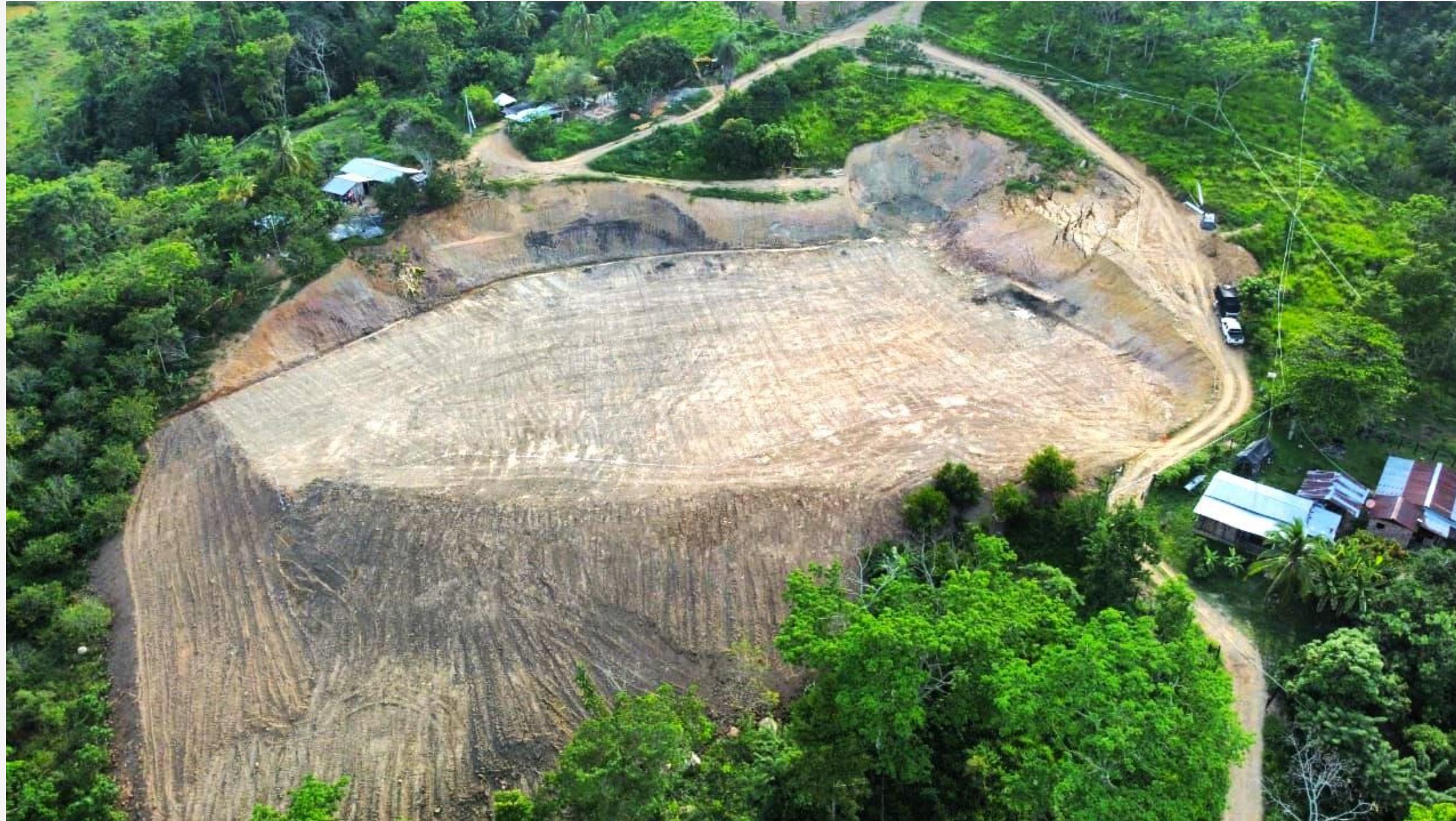
Aerial view of the project
