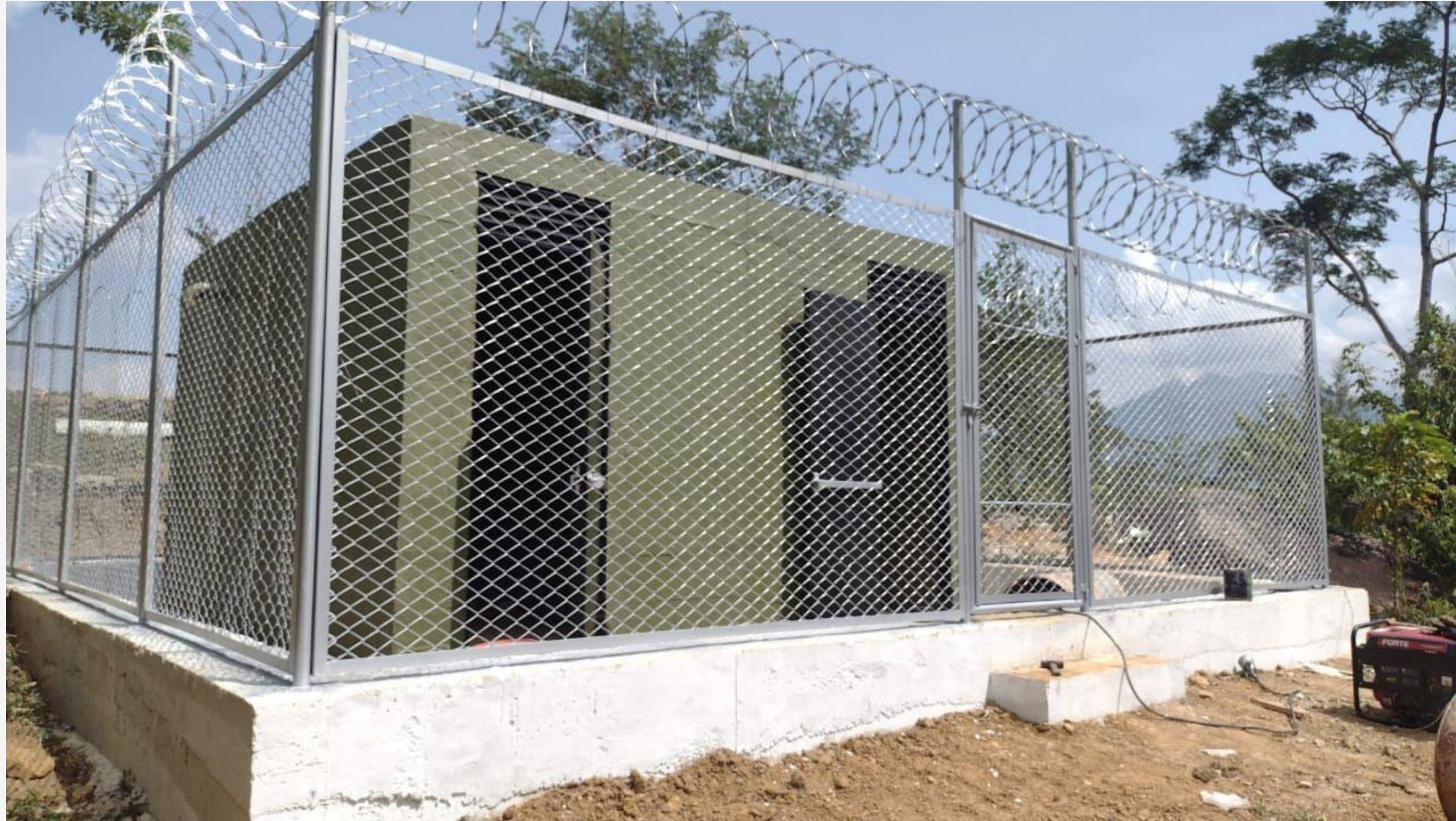
Completed - construction of the powder magazine
