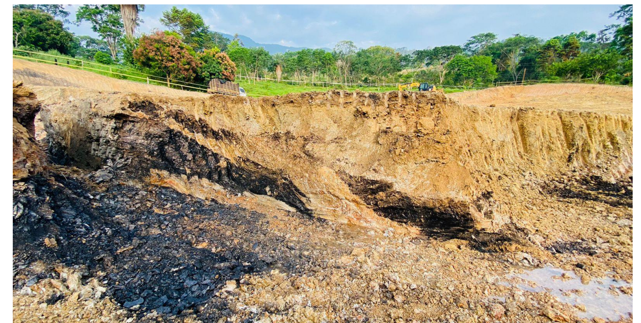
Terrace construction exposes coal seams at surface
