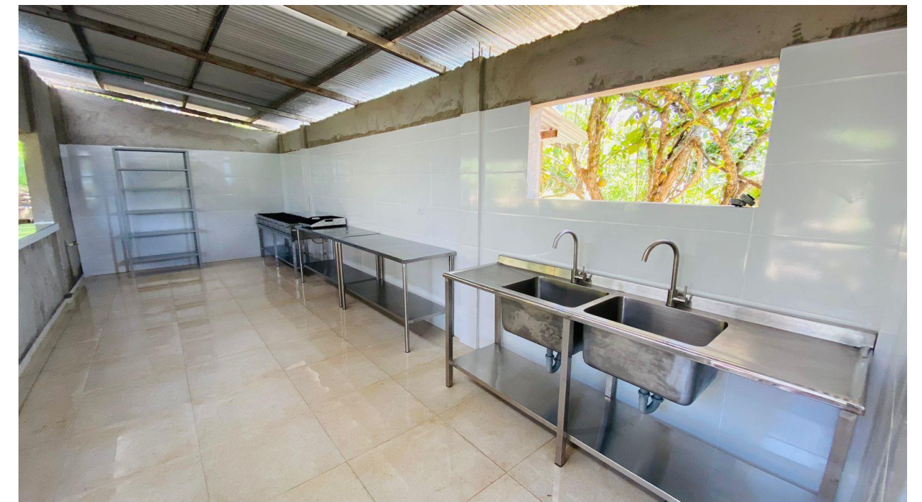
Camp kitchen construction
