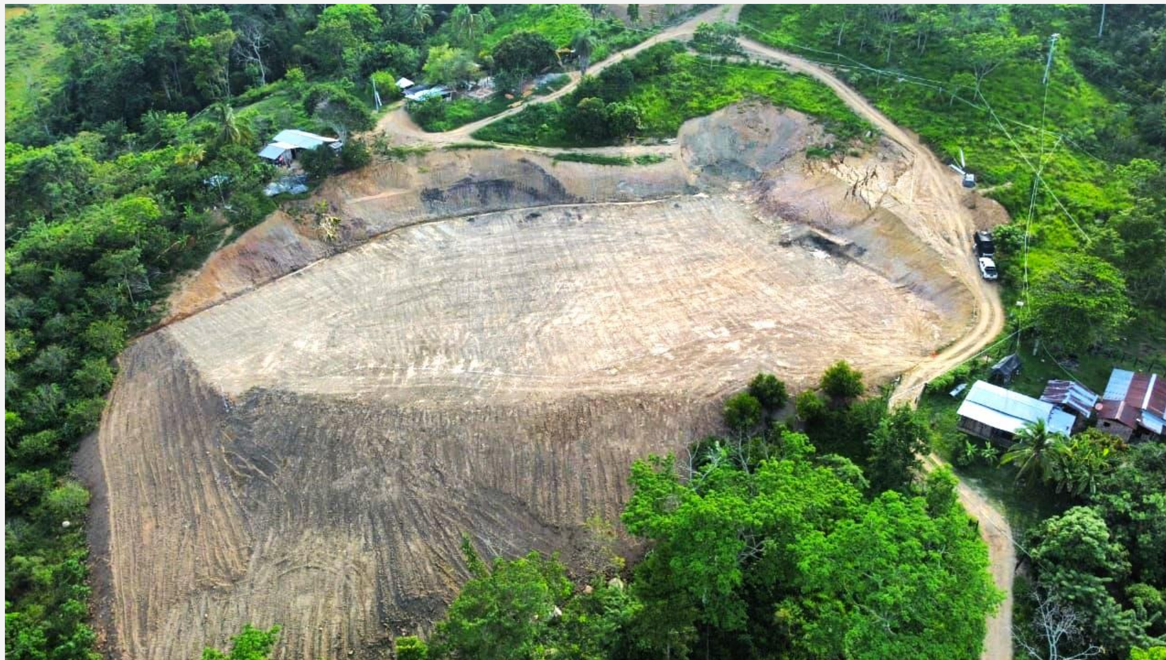
Aerial view of the project
